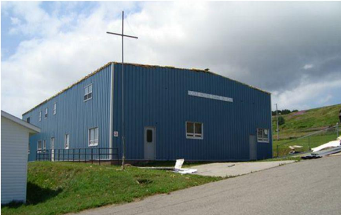
Figure 1: École Notre Dame Du Cap - View to West
